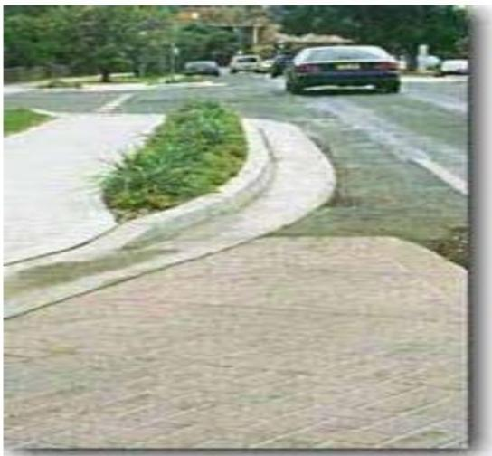
Figure 1.2: Application of Recycled Aggregate as Road Kerb (Source: Building Innovation & Construction Technology, 1999)
