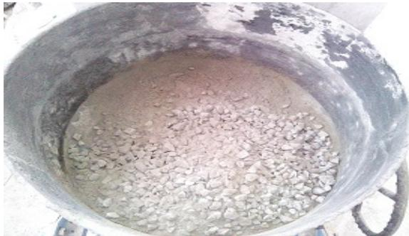
**Figure 3.1** Mixing of coarse aggregate and fine aggregate
